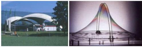
**Fig. 10: Concrete shell structure designed by Heinz Isler (left) and soap film experiment producing minimal surface (right) [20].**
