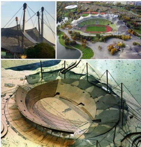
**Fig. 11: Munich Olympic stadium, Frie Otto, 1972. The Stadium makes extensive use of tensile roofing construction [25, 26]**
