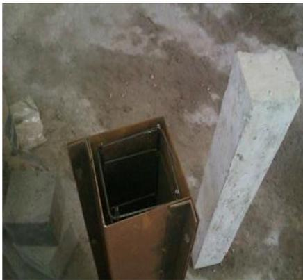
Fig.2 Concrete jacket before casting
