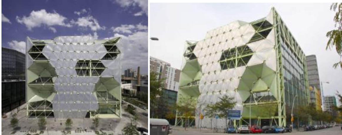
Figure(7): The main façade has a quilted appearance, owing to a sophisticated pneumatic system which lets in light or creates shade, according to the position of the sun, providing energy savings of 20%.
