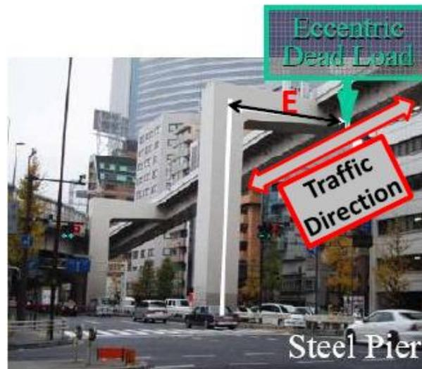
**Figure 2: Steel C-Bent Bridge Pier**
