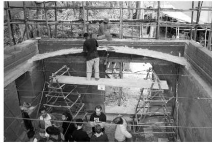
(B) The construction of the 1st floor vault is under process
