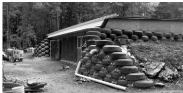
(B) exterior wall from tyres filled with rammed earth
