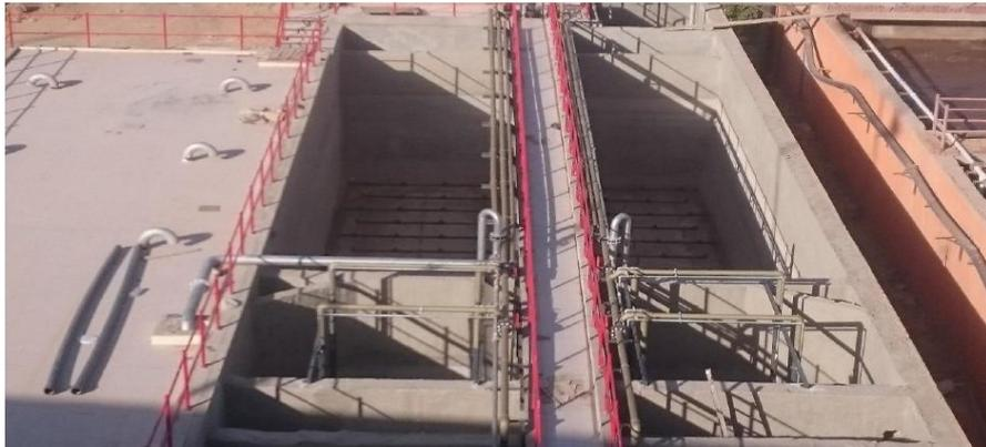
Figure 6. : Extended aeration air nozzles at W.W.T.P expansion (executed by researcher).
