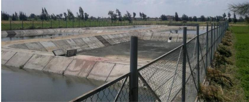
Figure 1. Quleaa SPO plant at Kafr ElShiekh , Egypt with 500m<sup>3</sup>/d capacity.
