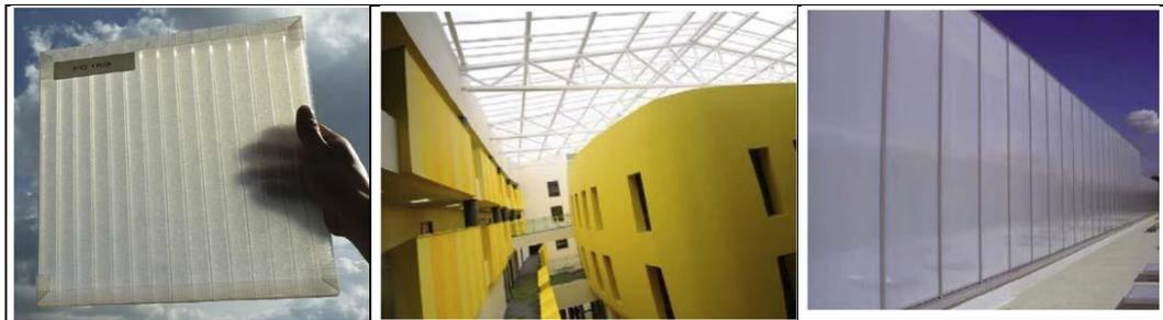
Figure 13: Application of aerogel-filled glazing panel on roof and walls of office building. (a) Aerogel-filled polycarbonate glazing unit; (b) Application on roof; (c) Application on wall <sup>(10)</sup>.
