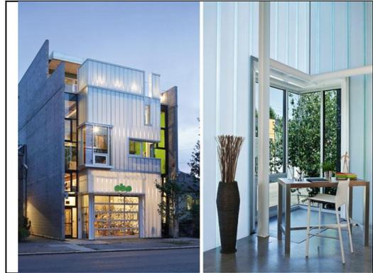
Fig. 10: Example of the application of aerogel in polycarbonate sheets in a multifunctional building in Seattle, Washington’s Fremont District <sup>(1)</sup>.
