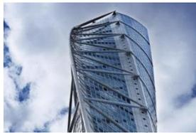
down through the height of the modules. The bottom slab of each module is a strengthened cantilever floor slab which supports the perimeter columns of the upper storeys in the module. While floor slabs are 27cm thick, strengthened cantilever slabs of modules that protrude from the core are 90cm thick at the cantilever root reducing to 40cm at the perimeter.
