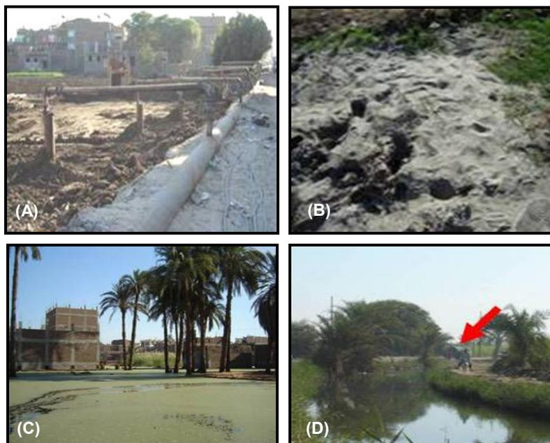
**Figure (2):** Field photographs showing: (A) water pumping during sewers net installation, (B): fine particles removed from the aquifer, (C) raw sewage overflows into streets (green color refers to algae cover), and (D) discharge of raw sewage into Qus irrigation canal.
