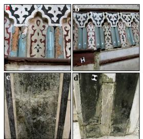
Figure (2) Shows deterioration phenomena of the mihrab <u>a</u>. breakdown of some ceramic units as peeling of the glaze layer, <u>b</u>. replacing the ceramic units with other wooden units, c. flaking of the marble surface, d. the use of cement in fixing some marble units and surface deformation
