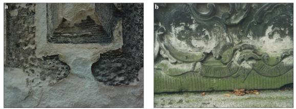
Figure (6) Shows <u>a</u>. architectural detail from Gotland sandstone, disintegration of stone under corrosive layers (*photo by the author*), <u>b</u>. fragment of the epitaph of Gottfried Mentzl and his wife Anna Rosina, disintegration of stone (sandstone with silica-loam sand binder) under the layers, action of salt and microorganisms (*photo by W. Domasłowski*)
