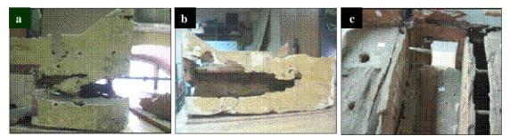
Figure (10- a, b, c) deterioration of wood (weakness in the bonding forces between fibers), and fungi infection.
