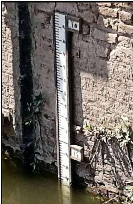
**Plate No. 36:** A Nilometer located at the eastern side of the front façade of the Bagouria barrage
