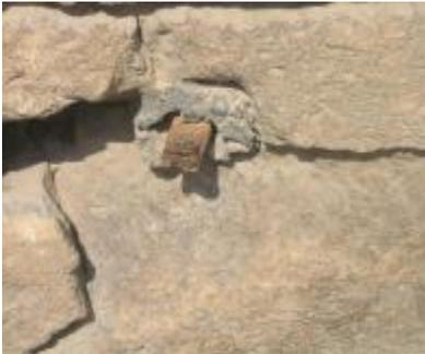
**Figs. 24- 27** The short iron bars which were used to tie blocks of alabaster veneers to the wall core and were fixed in walls with lead , the rusting and corrosion of hundreds thousands of caused expansion consequently produced forces which in turn created tension resulting in the 1<sup>st</sup> type cracks , also I have to cite that the alabaster veneer were felled by their own dead overweight .
