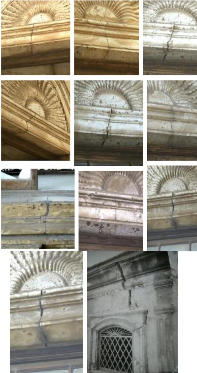
**Figs. 32 - 42** Display cracks of 2<sup>nd</sup> type in the springings of all lintels above openings in the mosque at positions of heavy load, the lower left photo. From Supreme Council of Antiquities archives (1935) .
