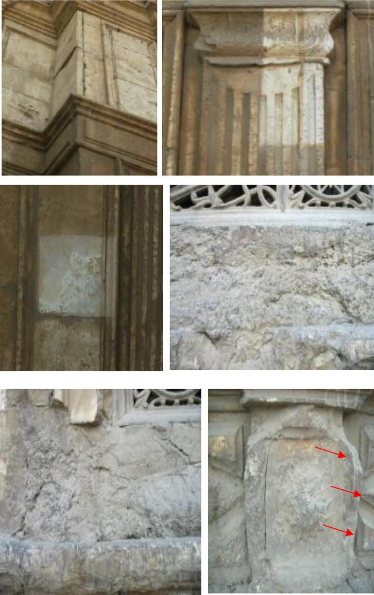
**Figs. 102-107** Muhammad Ali Mosque show that the soiling areas easily removed and another type of soiling is not easily removed , also here there is a thick black crusts of irregular shape or discoloration (soiling) to crust are just an extreme case of the lower right photo , Since such crusts are brittle and tend to detach from the alabaster (red arrows) .
