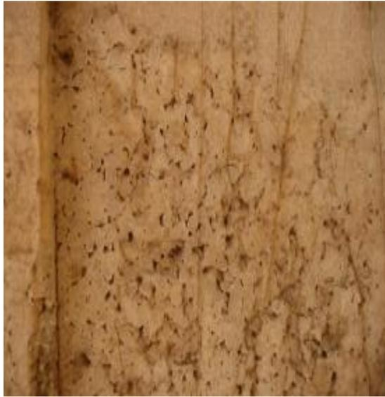
**Figs. 74-75** Display superficial coarsening and granulation on the surfaces of the travertine of chapels at Karnak smoothed by corrosion polishing as external deterioration factors.
