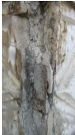
**Figs.165- 167** display some Man-made faults (erroneous restoration) in Muhammad Ali Mosque alabaster veneers were compensated with unsuitable material (Portland and white cement) and in with out character style .
