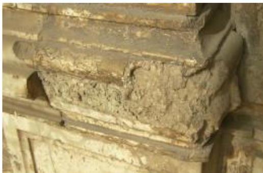
**Figs. 148-149** Display Back weathering due to loss of scales where is observed in Egyptian alabaster surfaces of both chapels at Karnak (above) Muhammad
