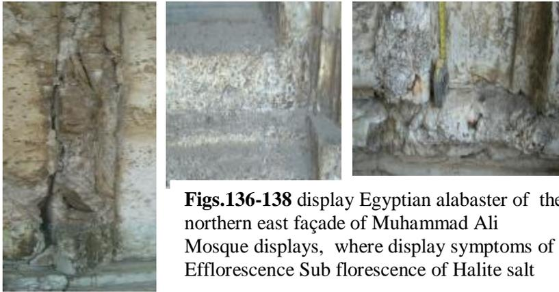
**Figs.136-138** display Egyptian alabaster of the northern east façade of Muhammad Ali Mosque displays, where display symptoms of Efflorescence Sub florescence of Halite salt
