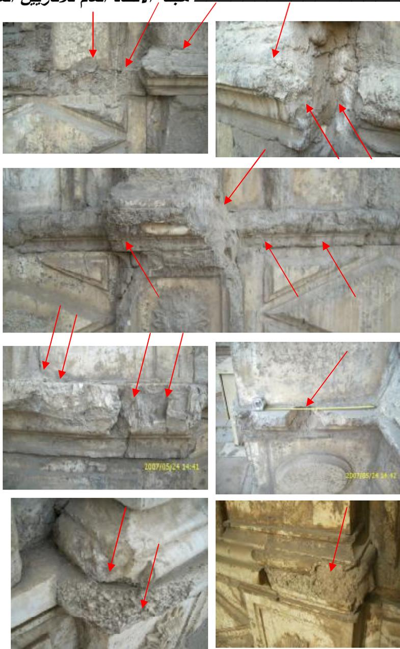
**Fig.48-54** Frailty and debility structure of some ornamental architectural elements of Egyptian alabaster of Muhammad Ali Mosque such as the Cavetto Cornices , in addition to being hanged partially on space , have exposed them to fracture and loss or to erosion (arrows) , also disintegration and soiling can be noted .
