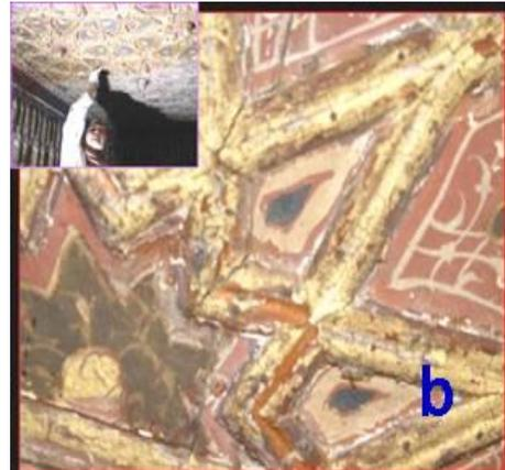
Fig. 11 a,b Photographs (macro and micro) corresponding to the gilded ceiling of El-Sadat house shows its status.( Notice the gilding craquelure).
