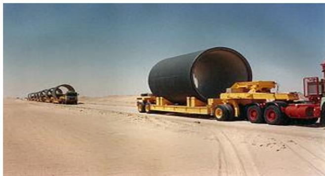
**Fig. 3. the transport of pipe segments for the artificial “Great River” in Libya.**
